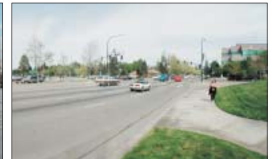
Poor Pedestrian Links
