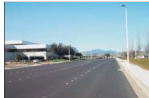
Roads are too wide
